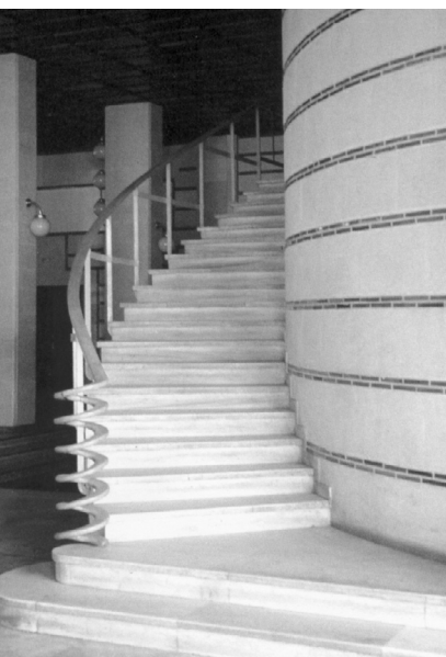
Figure 6 Stair detail, Faculty of Languages building.
