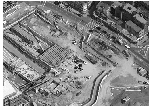
the site with the tunnel in the process of being covered
