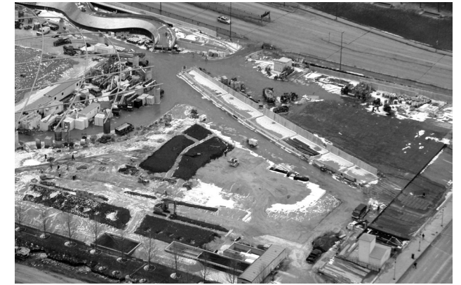
the Lurie garden under construction
