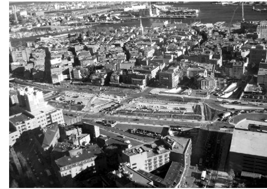
North End Parks under construction
